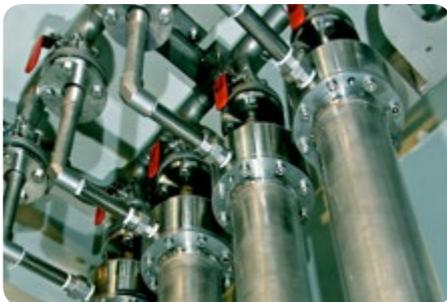
At first, raw biogas includes 48 to 65 % methane ( $\text{CH}_4$ ) as well as 35 to 52 % carbon dioxide ( $\text{CO}_2$ ) and low percentages of other trace gases which are seen as pollutants. Before the gas is fed into the natural gas supply network, the methane has to be separated.
